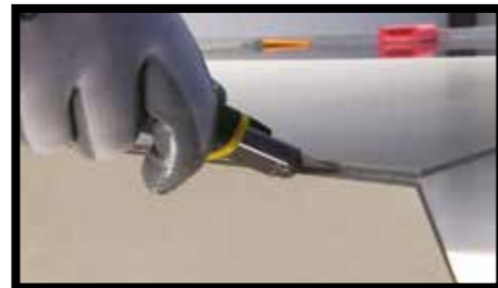
Fig.4 - For ZERO.3 3PLUS and ZERO.3 5PLUS, once the tile has been scored and the tile split, the cutting process is completed by cutting the fibreglass with a common cutter.
