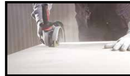
Fig. 7 - All versions of ZERO.3 can be cut using diamond discs fitted onto hand-held electrical grinding machine. Disc rotation speed must be high (>10000 RPM) and a low feed rate (< 1 m/min). Depending on the type of disc and the length of the cut, it may be necessary to cool the disc with water. Recommended discs are the thin types generally used for cutting porcelain stoneware. The advantages of this type of cut include ease-of-execution and the possibility to cut during installation.
