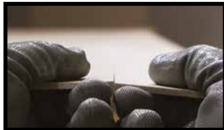
Fig.3 - After scoring, it is sufficient to bend the slab to detach the two pieces.
